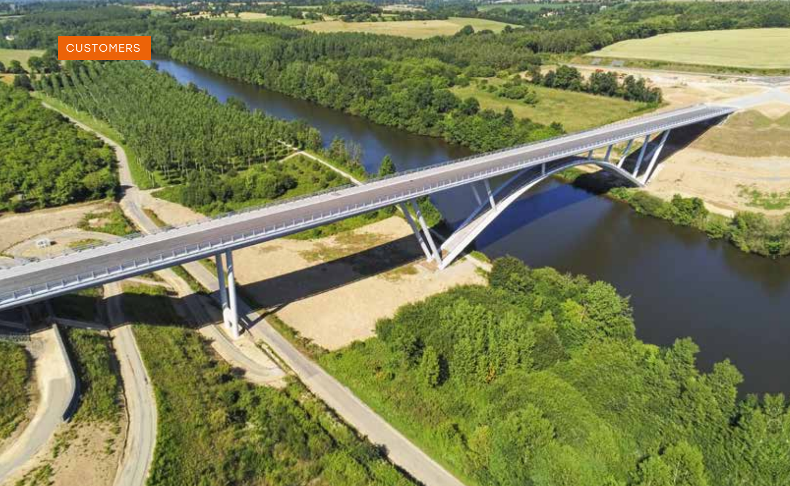
Key to the success of the Château-Gontier bypass project, the Mayenne viaduct opened to traffic in October 2022
