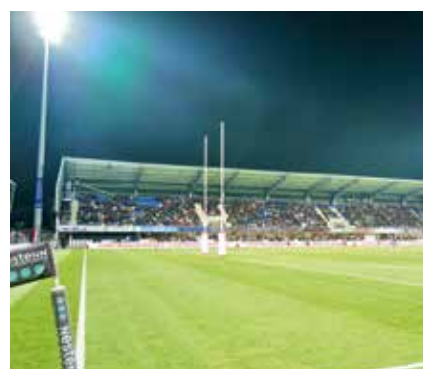
Design & Build The east stand of the Rabine stadium in Vannes was delivered two weeks ahead of schedule in December 2022
