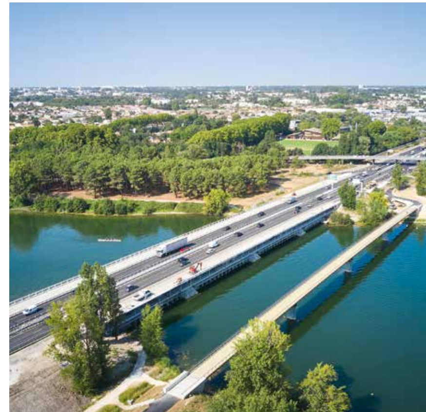
▼ Upgrading the Bordeaux ring road to 6 lanes was essential to ease traffic congestion across the city
