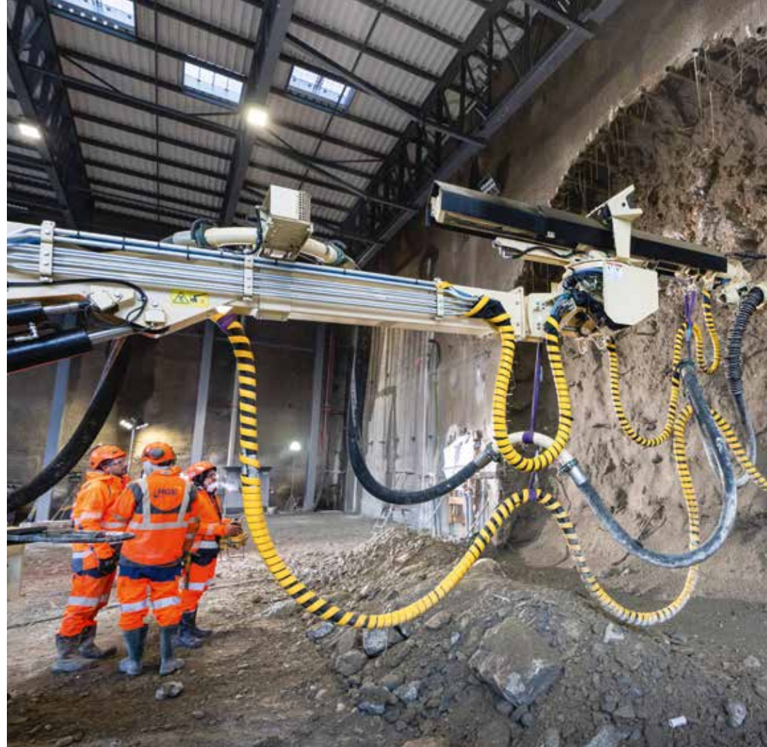
Work begins on the French entrance to the Lyon-Turin rail tunnel
