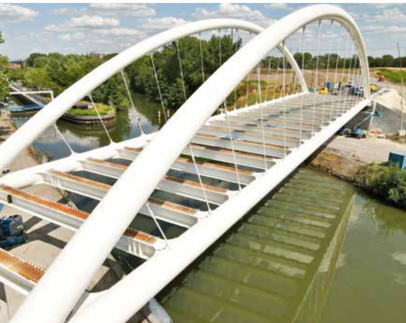
▼ The Valenciennes bypass is facilitating mobility by removing city centre congestion. This is the bowstring bridge river crossing
