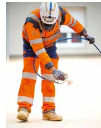
▲ NGE has developed a paint to reduce the effect of urban heat islands
