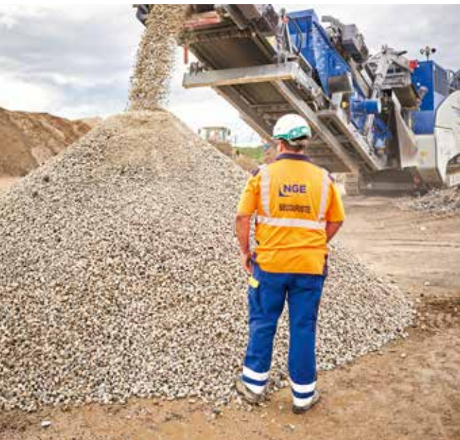
▼ Concrete crushing at the Martignas-sur-Jalle worksite waste recovery centre
